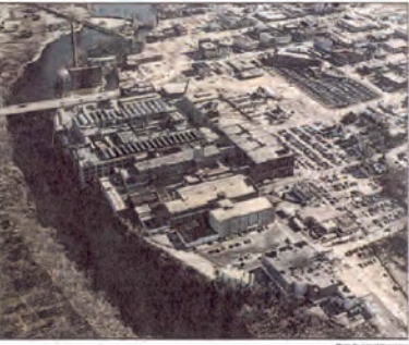
This overview of the 43-acre Uniroyal site on the St. Joseph River in Mishawaka was photographed several years before the last building on the site was closed in 1977. The photo was in files at Mishawaka City Hall when the city selected the Troyer Group to replan it.
