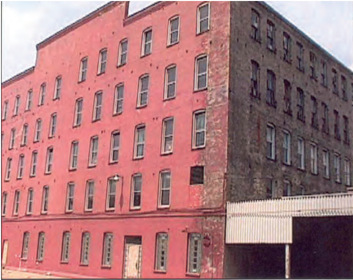
Former Woolen Manufacturing Company building.
