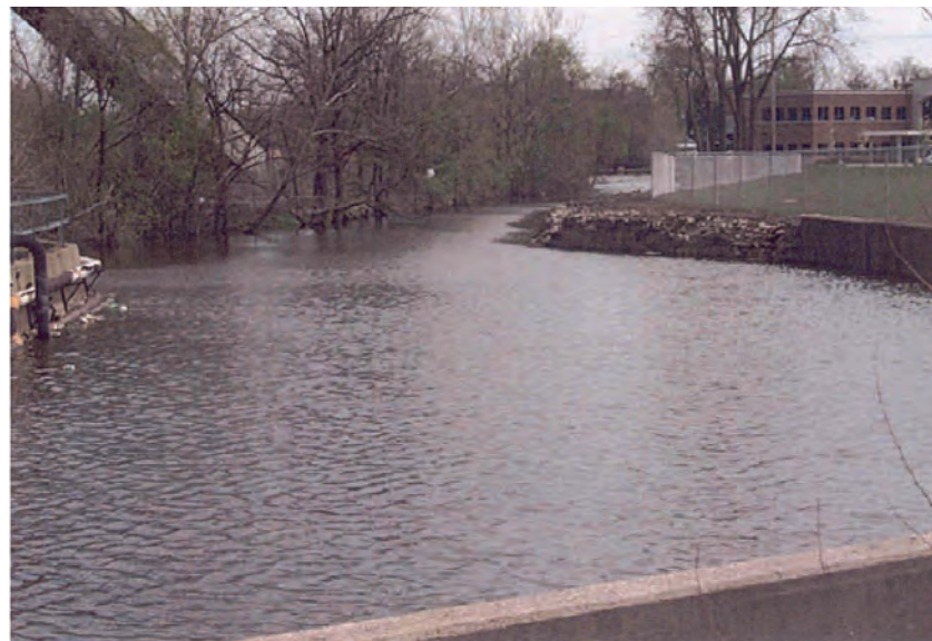
View of existing race looking east toward the dam.
