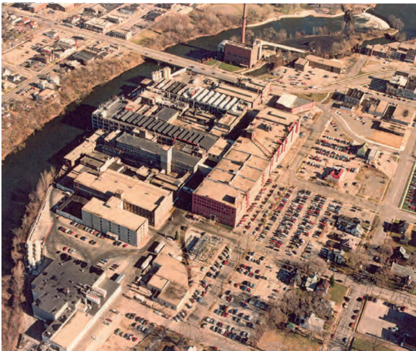
View of project area looking from the southwest.
