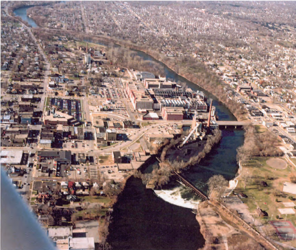
View of project, river and central business district looking west.
