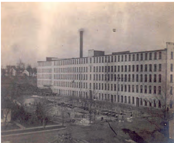
Building under construction at Mishawaka Woolen Manufacturing Company
