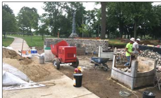
Veterans Plaza construction
