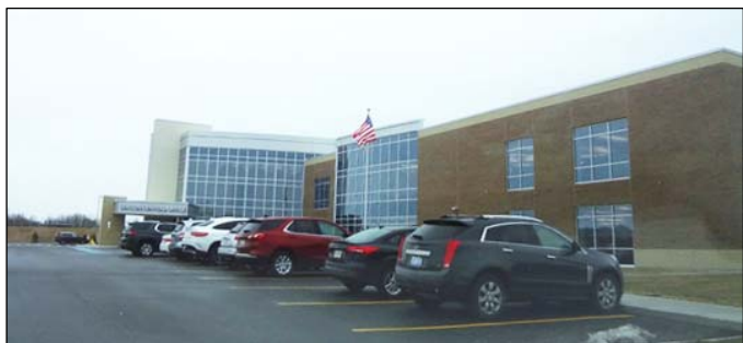
Beacon Administrative Facility, February 2020
