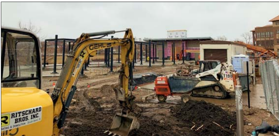
Biergarten under construction, February 2020
