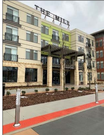
The Mill – North Entry & Leasing Area
