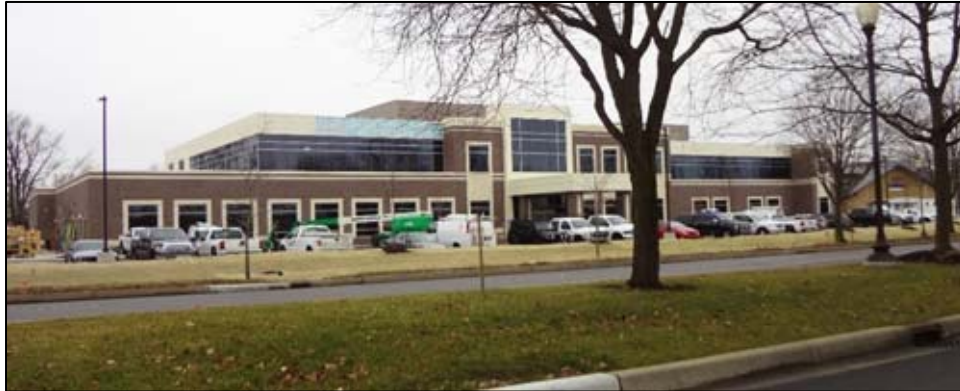
Vibra Hospital nearing completion, February 2020
