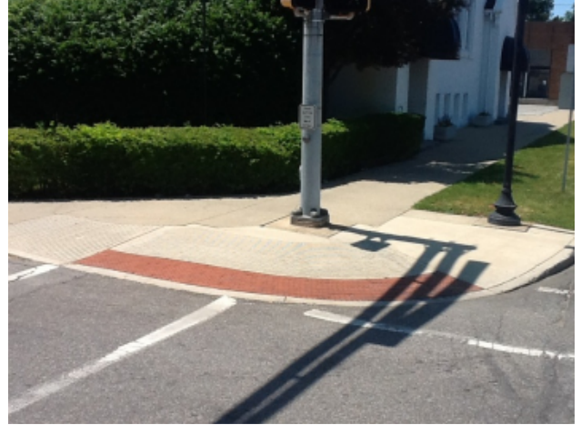
Lincolnway and Spring St. (Photo Illustrates proper location of detectable warning along full width of flush connection. Note that truncated domes have been sheared off and no longer serve intended purpose. Crosswalk should encompass entire flush connection.)
