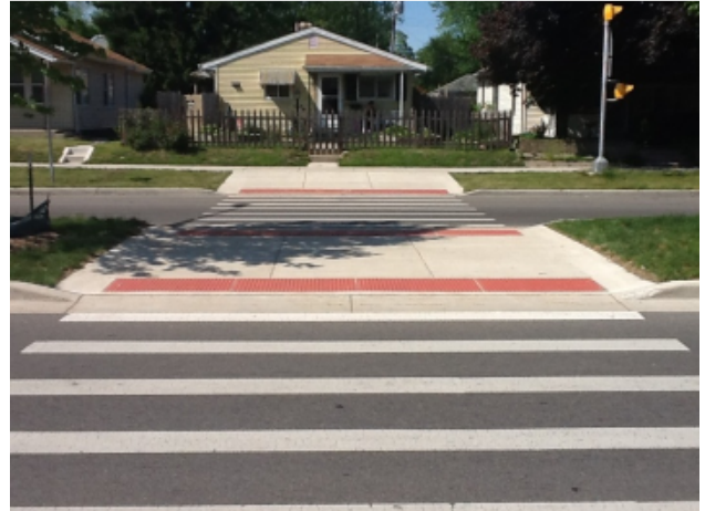
Mid-Block Crossing at Milburn (Photo illustrates detectable warnings full width and depth at refuge island and located wholly within crosswalk)
