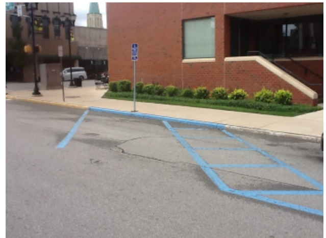
Photo illustrates on-street angled parking on Main St. Access aisle provided but not connected to accessible route. Signage mounted below 80" adjacent to a pedestrian circulation area.
