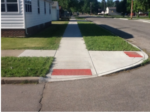
11 th St. and West St. (Photo illustrates proper use of flares for two ramps on tight radius, however, detectable warnings are not full ramp width.)
