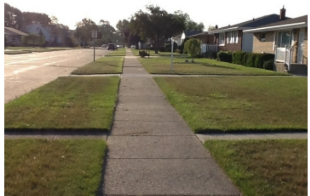
Photo: Example of 5’ sidewalk width (W. Eleventh Street between Wells and West St.)
