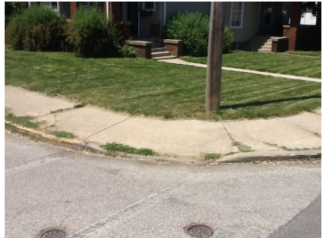
7 th St. and Main St. (Photo illustrates common issue in older neighborhoods. No detectable warnings, no landings, non-compliant cross and running slopes. Utility pole location complicates solution as potential obstruction.)
