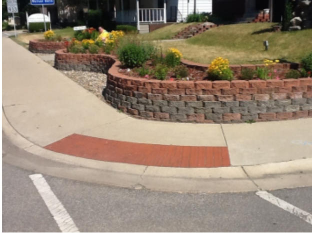
Lincolnway and Columbia St. (Photo illustrates typical case where no landing exists due to ROW limitation or other physical constraint.)
