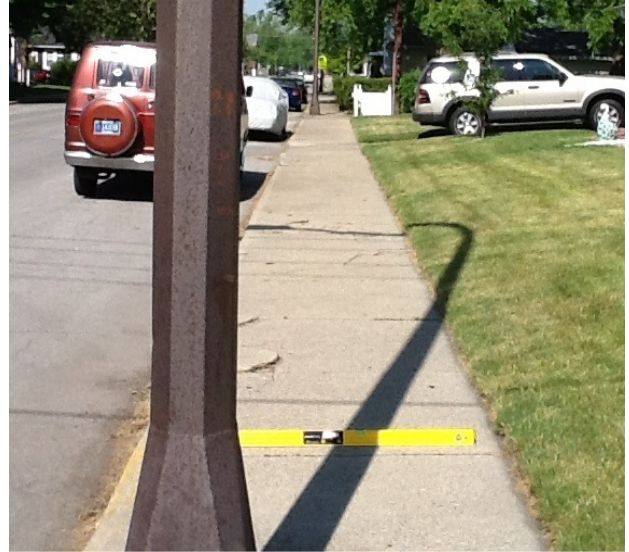
Example of Utility Obstruction narrowing sidewalk width to under 48" minimum required (E. 3 rd St. between Home St. and Alford St.)
