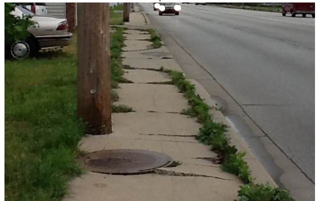
Photo: Example of ground plane utility conflicts as displacement and slip/trip hazard (Union St. between 11 th and 12 th St.)
