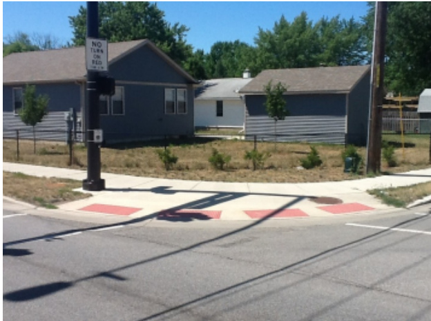
McKinley Ave. and Division St. (Photo illustrates common misuse of detectable warnings. Warnings to extend entire width of area flush with street. This provides gaps which could be missed by pedestrian with low vision.)
