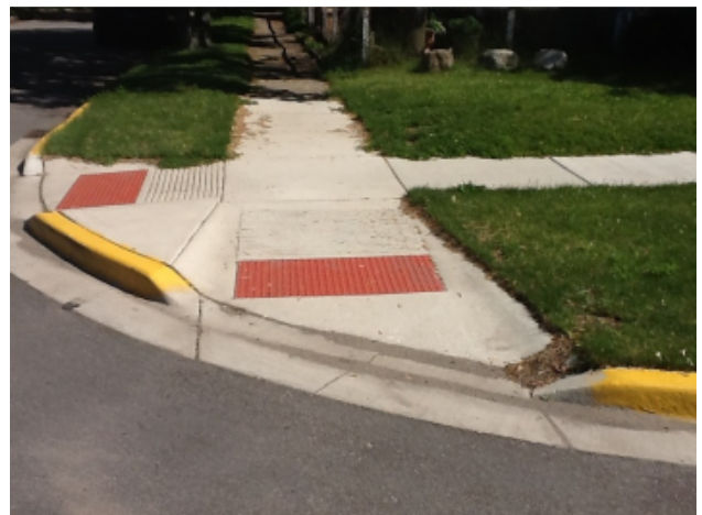
Geyer Ave. and Milburn Blvd. (Photo illustrates common misuse of flares. Flare to lawn is not necessary. Inner flare is too steep creating trip hazard.)
