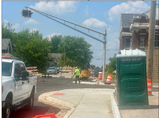
Signal and Storm System Improvements at Main St. and Eighth St.
